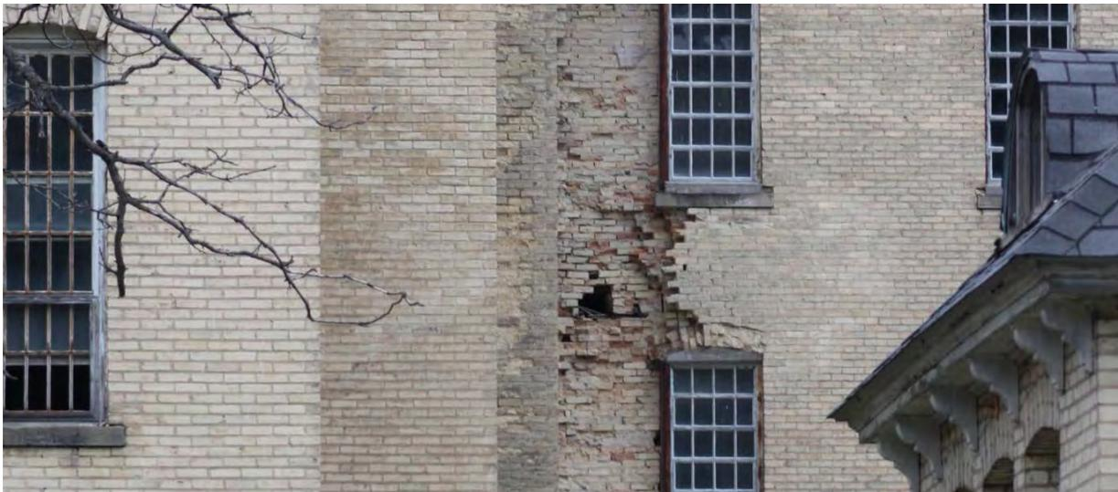
**Wall showing damage where water has concentrated. This kind of damage can often be prevented by sloping the ground away from the building and using effective gutters and downspouts.**
