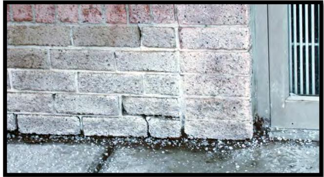
**Bricks near roof run-off or broken downspouts.** These areas receive concentrated levels of water. They often show staining and have higher levels of moisture. Brick and/or mortar damage can often be found in these areas.
