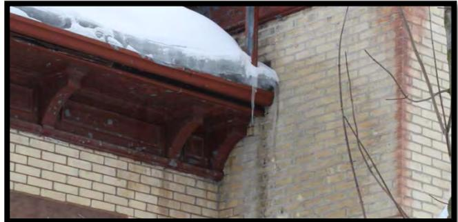
**Buttresses.** Some older brick homes have thickened structural brick posts that stick out from the building. These are especially common in remodeled churches and warehouses. Buttresses are exposed to the wet and cold from three sides and receive less heat from the interior.
