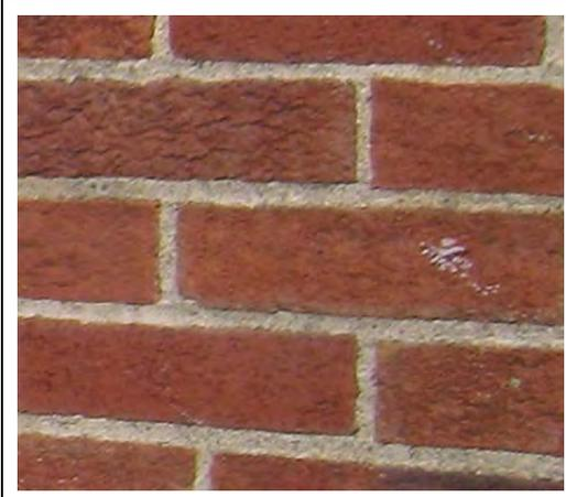
**This wall has been exposed to water and multiple freeze-thaw cycles, but shows no sign of damage.**
