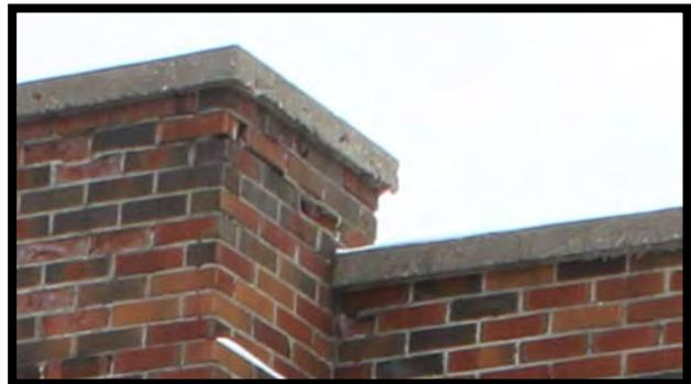
**Chimney.** Most older masonry buildings have an exterior chimney made of the same masonry as the walls. Above the level of the roof, this brick is exposed to weather and receives little heat from the interior for drying. In older buildings, the chimney is often replaced or removed due to freeze-thaw damage.
